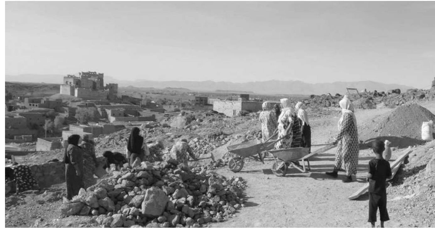
Worksite, Ourika, Morocco
