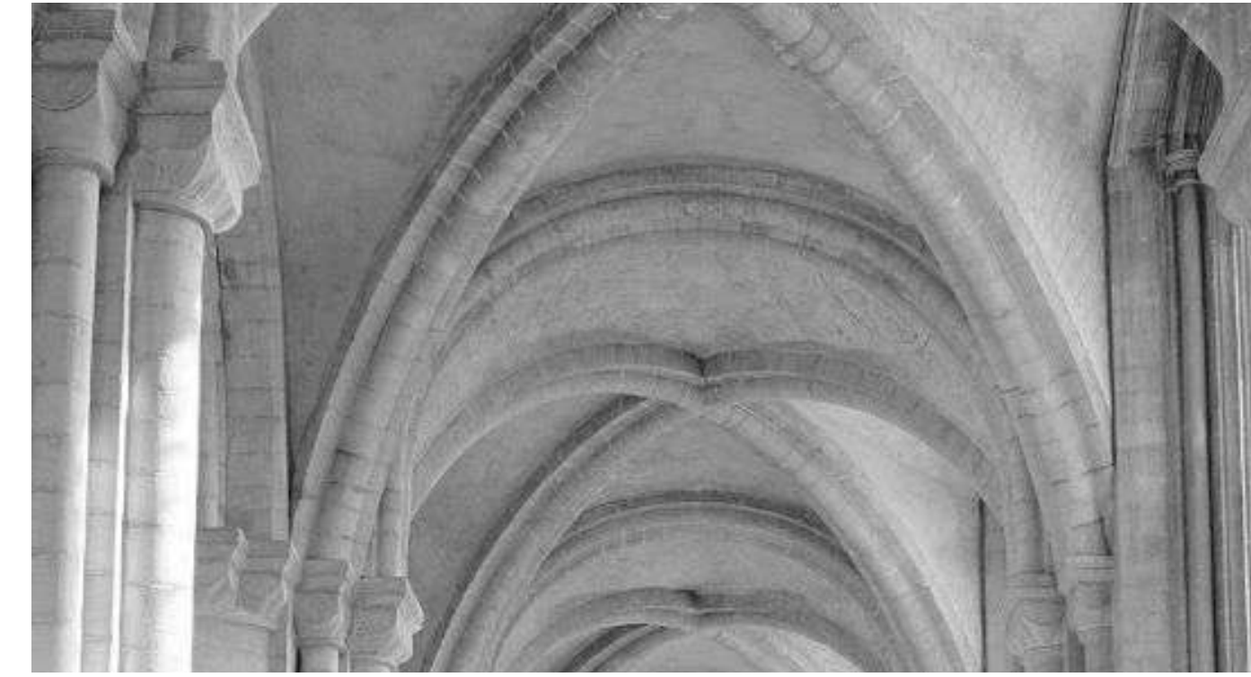
Romanesque rib vaulting, Peterborough Cathedral (begun 1118) south aisle.
