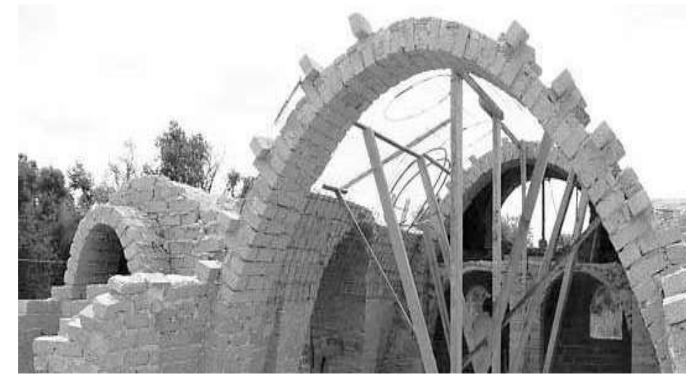
Geography : Mexico Climate : Subtropical Community : - Construction technique: Pumice blocks Period: 21st
